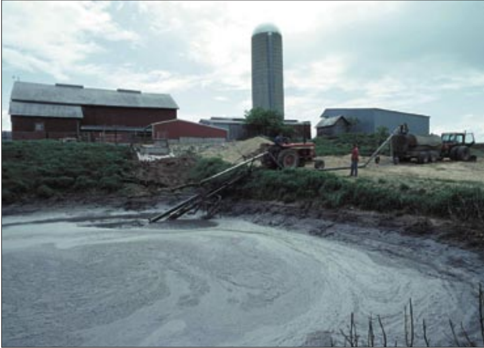
Liquid Manure Storage Pit at a Dairy in Northeast Iowa (IOWA USDA NATURAL RESOURCE CONSERVATION SERVICE)
