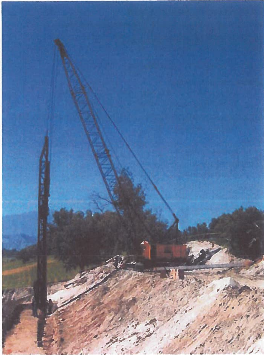
PHOTO 1 Pile Driving Rig
