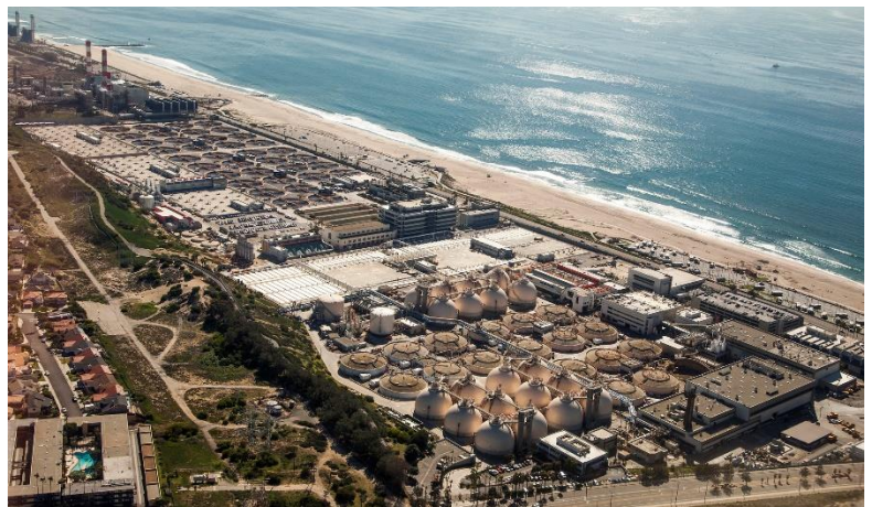
The Hyperion Water Reclamation Plant, which has been operating since 1894, is Los Angeles' oldest and largest wastewater treatment facility. In July 2021, it spilled 17 million gallons of partially treated sewage into Santa Monica Bay.
