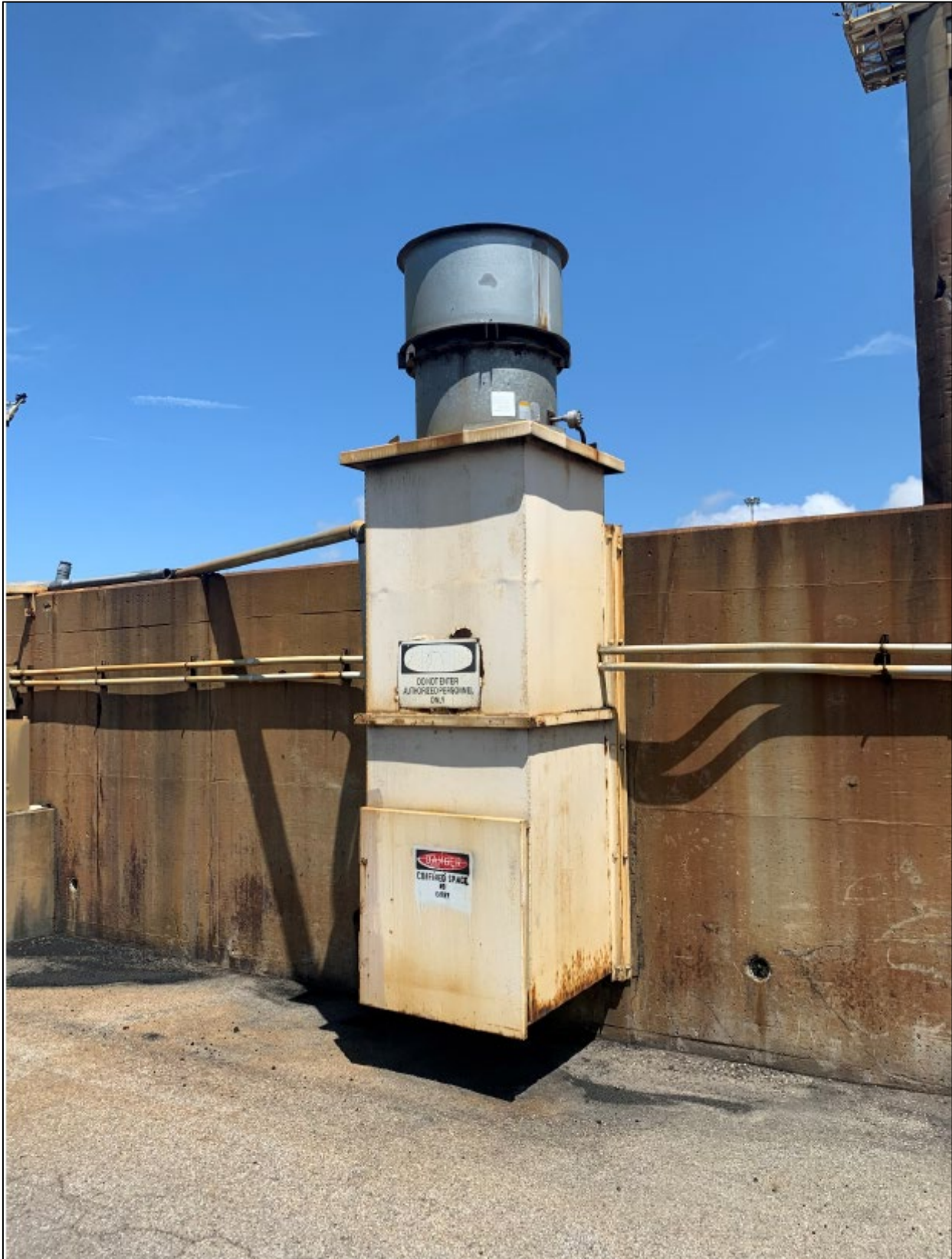
Figure 2.4.1. South Reclaim Tunnel exhaust as seen on July 9, 2020.
