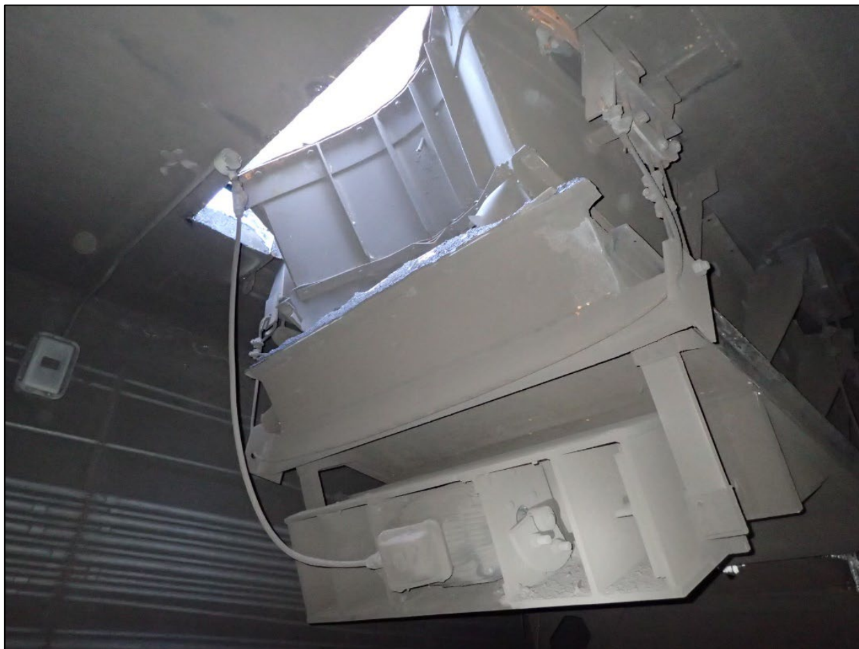
Figure 6.3.2. Feeder 21 from beneath the feeder hole, in the North Reclaim Tunnel.
