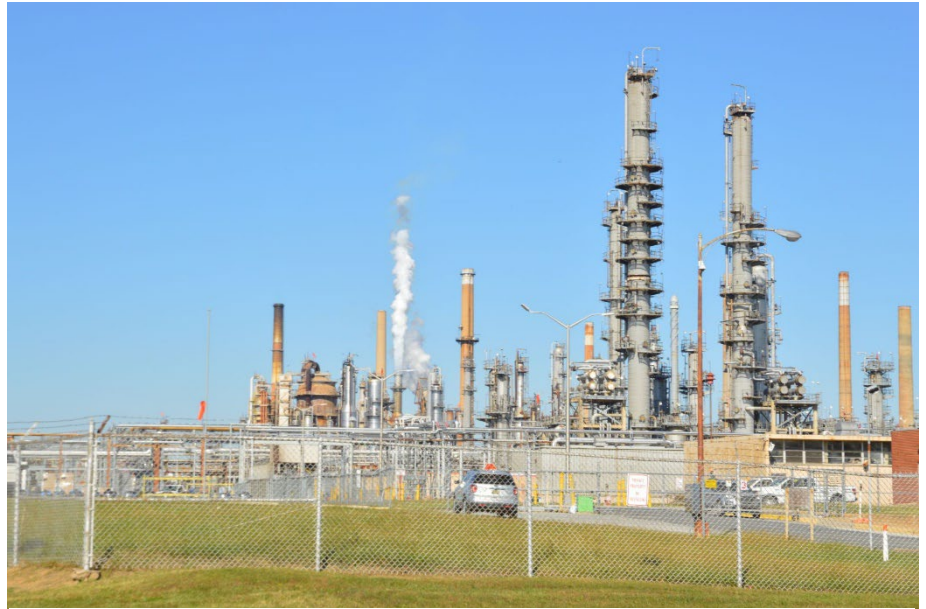
The law directs EPA to review wastewater treatment standards for refineries and other industries ever year, and at least every five years. But EPA has not updated the standards for refineries since 1985.
