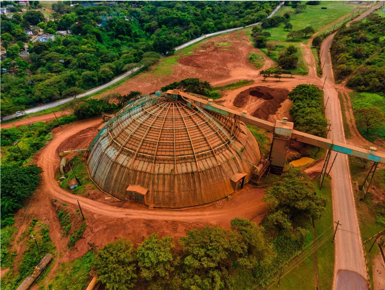
A bauxite storage facility at the Discovery Bauxite plant in Discovery Bay, Jamaica, where bauxite is transported via rail from inland mines to be shipped overseas.
