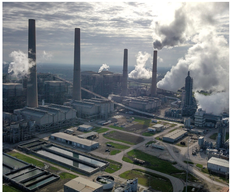
The Petra Nova carbon capture and storage project, southwest of Houston, is one of the largest in the world. It collects carbon dioxide from the burning of coal at the W. A. Parish power plant and pipes the carbon underground for injection into aging oil fields, to increase oil output. The system restarted in September after being shut down for more than three years.
