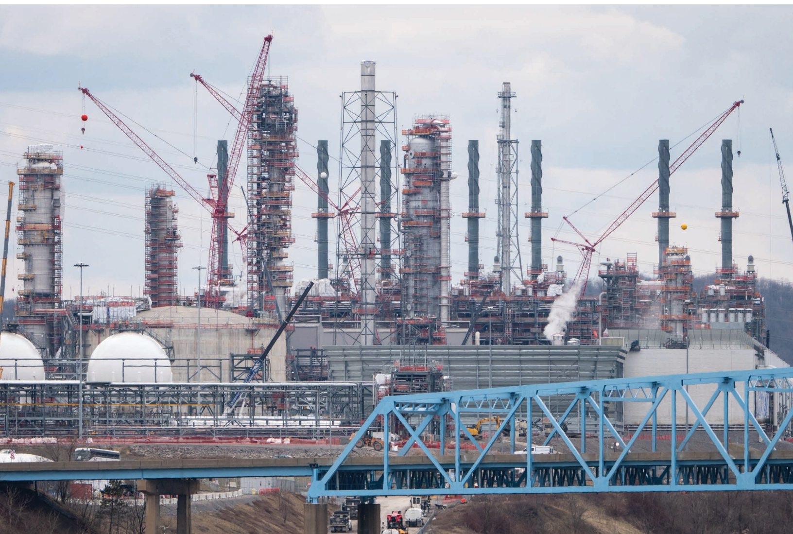
The Shell Monaca ethylene and plastics plant under construction northwest of Pittsburgh. Photo by Mark Dixon, Flickr.
