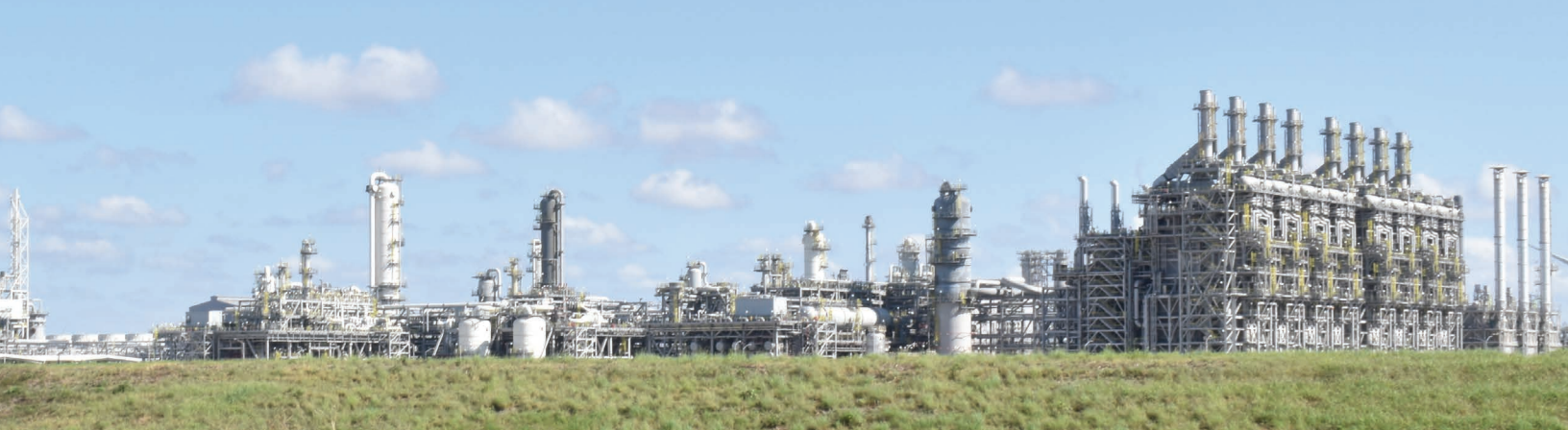
Gulf Coast Growth Venture's ethane cracker furnaces used for ethylene production on the right, distillation towers center, and to the left, the facility's monoethylene glycol (MEG) unit.
