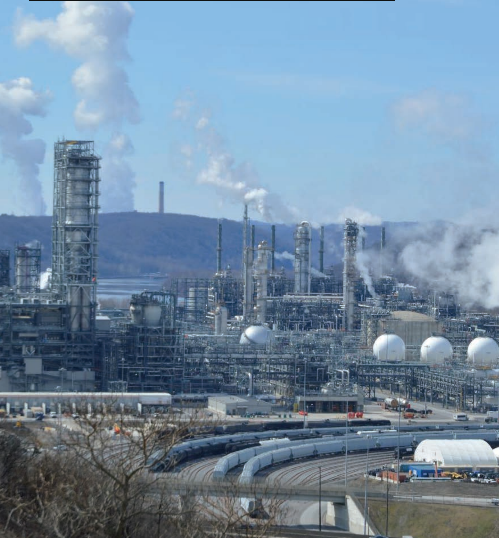
Smokestacks and emissions from the Shell Monaca plastics plant in Pennsylvania.
