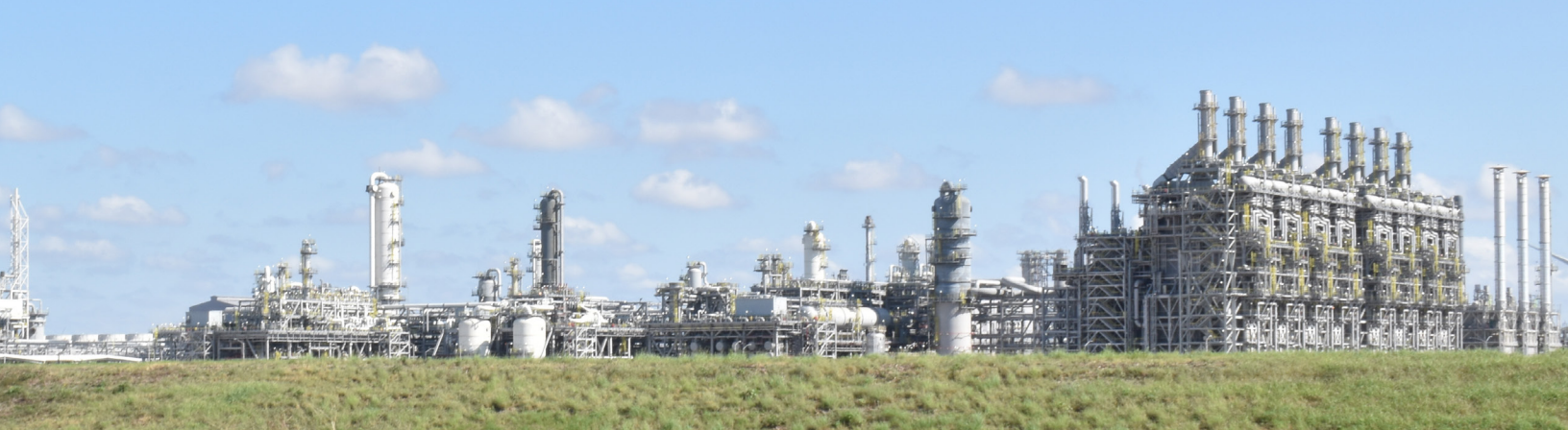
Gulf Coast Growth Venture's ethane cracker furnaces used for ethylene production on the right, distillation towers center, and to the left, the facility's monoethylene glycol (MEG) unit.
