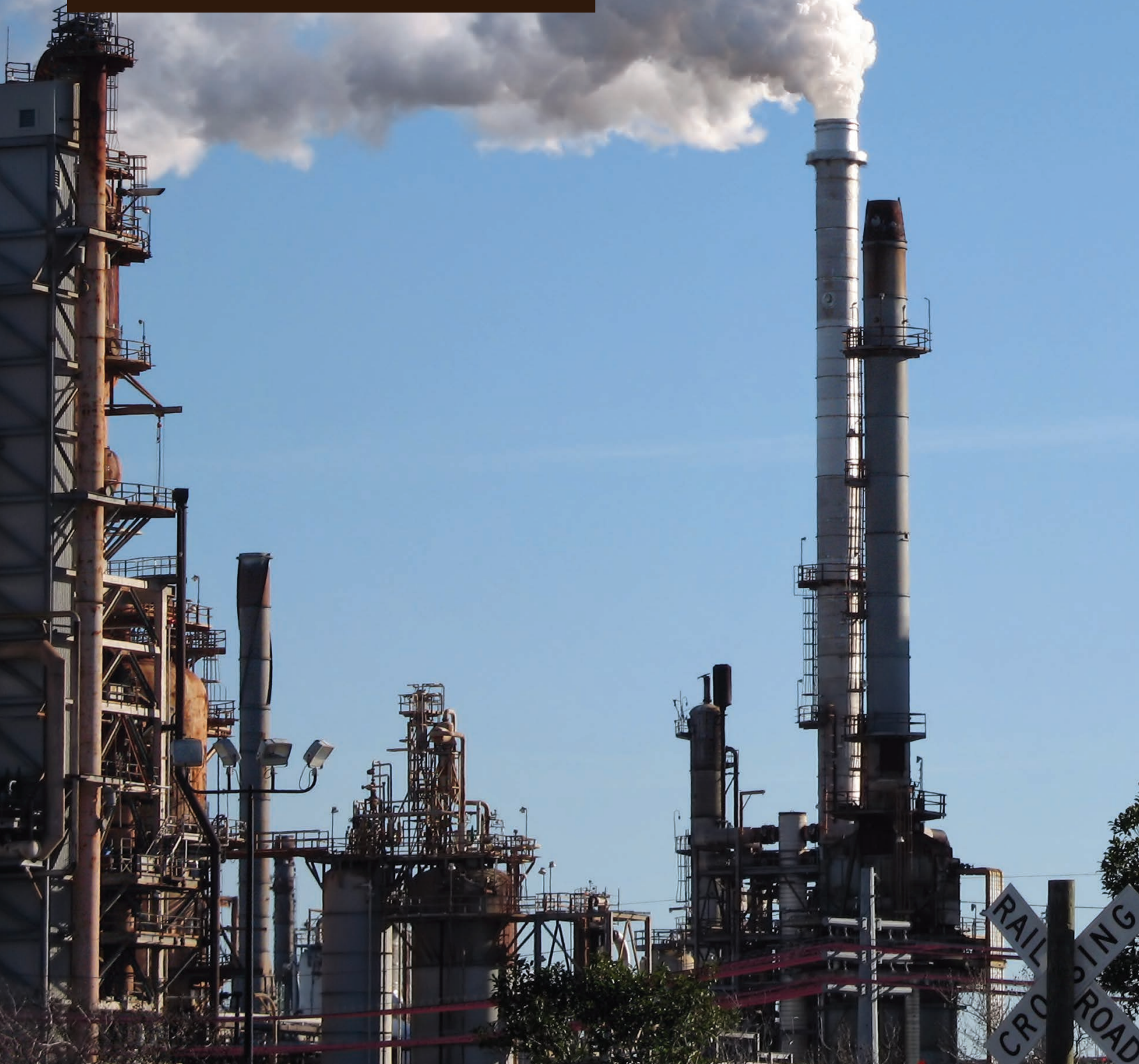
The Chalmette Calcining Plant in Louisiana processes petroleum coke for use by industry.
