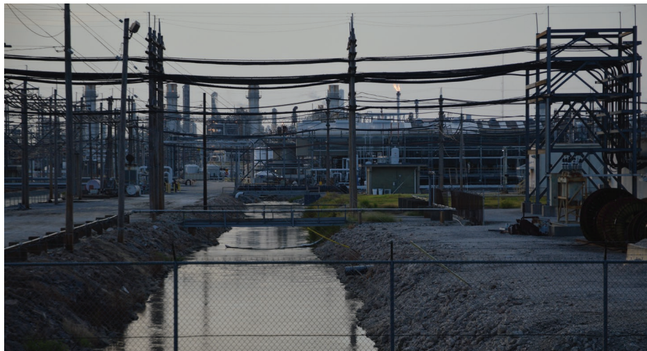
EPA has not updated its wastewater treatment technology standards for the plastics industry in 31 years. Pictured here is a drainage ditch at the Dow Plaquemine chemical plant in Louisiana.
