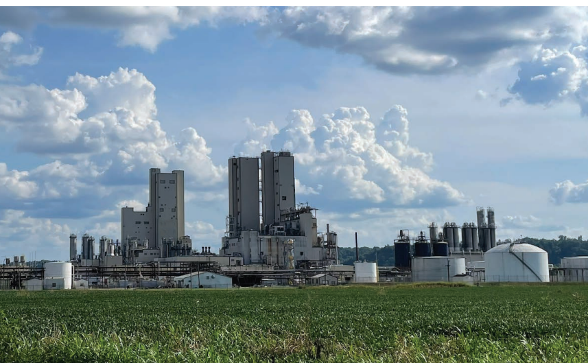
The APG Polytech plant in Apple Grove, West Virginia. Photo by Beyond Petrochemicals.
