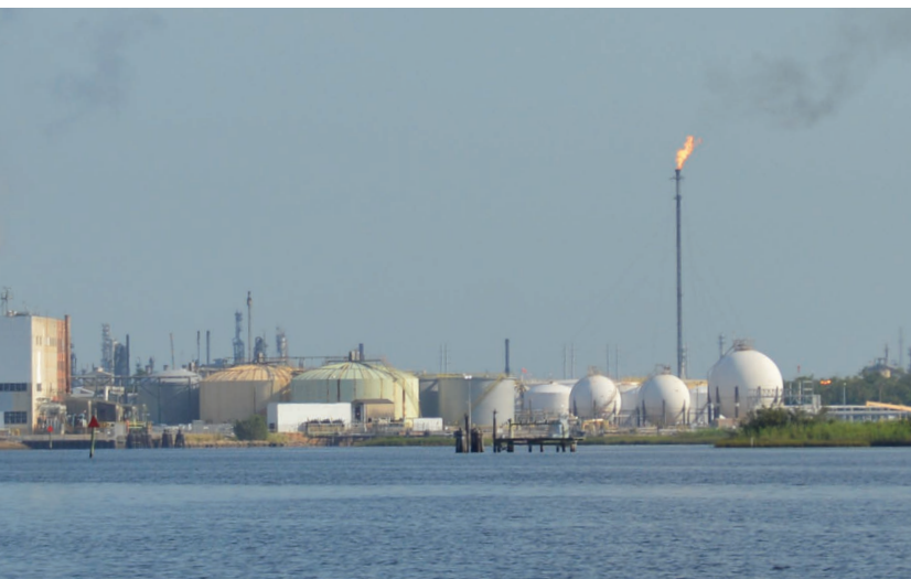
The Westlake Eagle US 2 Lake Charles plastics chemical plant released 83 million gallons of wastewater a day into the Calcasieu River in 2023.
