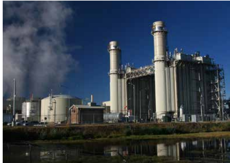
The growth in gas power plants for data centers could mean an increase in demand for natural gas of 6 billion cubic feet per day by 2030, which would also mean more pipelines, processing plants, leaks and greenhouse gas pollution. Photo by Arbyreed, Flickr.
